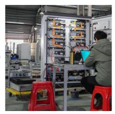
MOTOMA solar energy storage italiation in Sudan, using dual hybrid inverte and six M90 PRO lithium batteries. Learn how this nearly 100kWh solar storage systems setup delive ...
